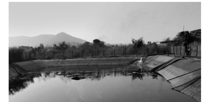
A farm pond has been created serving as a reservoir for harvested rain water, this water is being used in cooling towers and gardening
